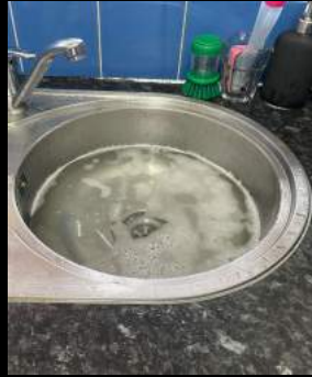
28 SEVERELY CLOGGED SINK
